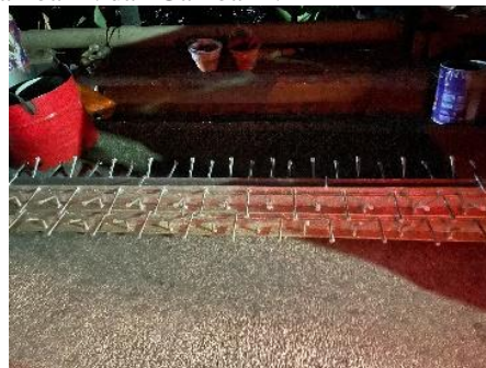
Gambar 2. Sambungan Tipe Strip Seal
